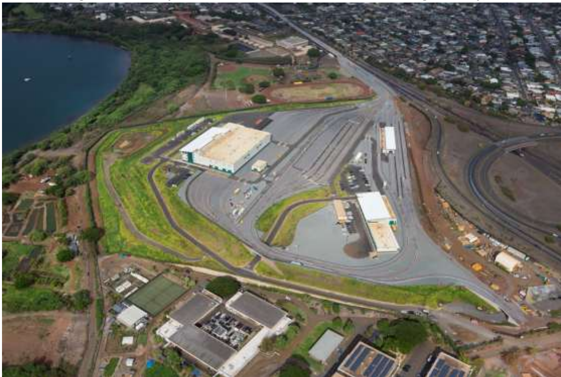
Figure 3.3 Rail Operations Center (Maintenance and Storage Facility)
