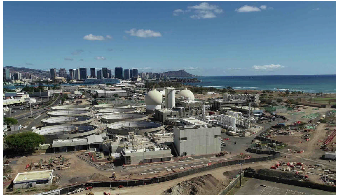
Sand Island WWTP
