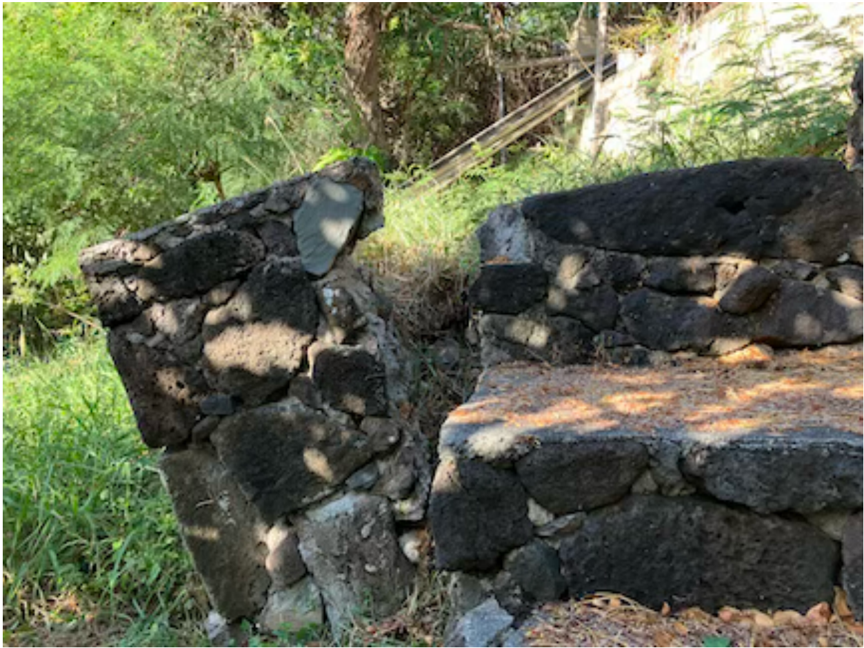
Photo 2 caption: This permitted rock retaining wall is about 30 years old but showed no sign of leaning when we purchased the property in 2010. A haole koa tree at the far end is probably preventing it from falling totally over.
