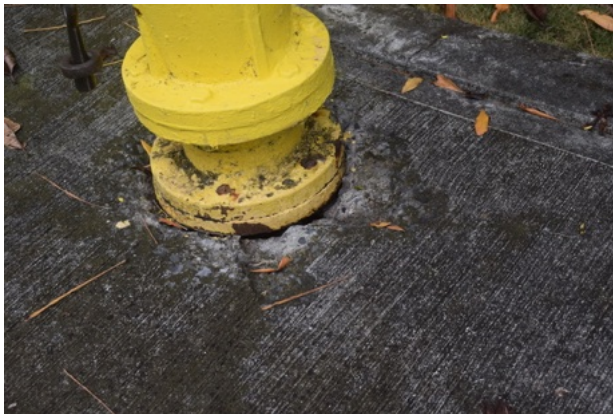
Fire hydrant busting through a substantial Concrete foundation
