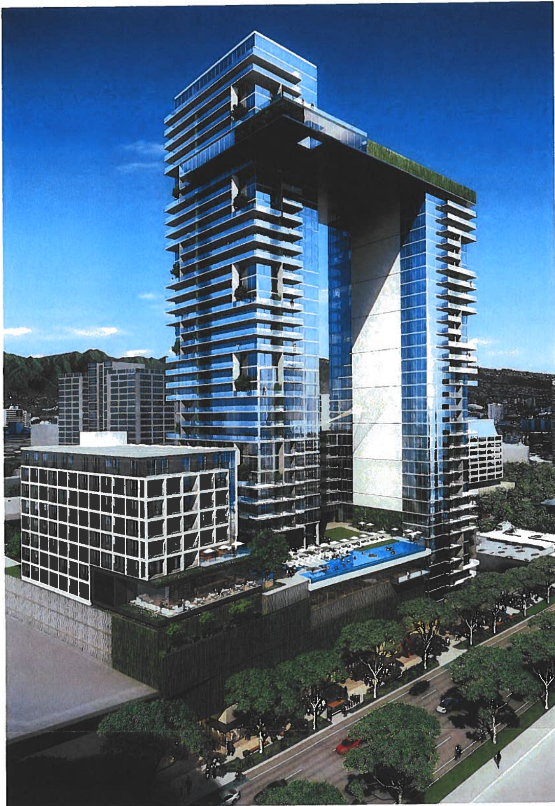
VIEW FROM SOUTHWEST
