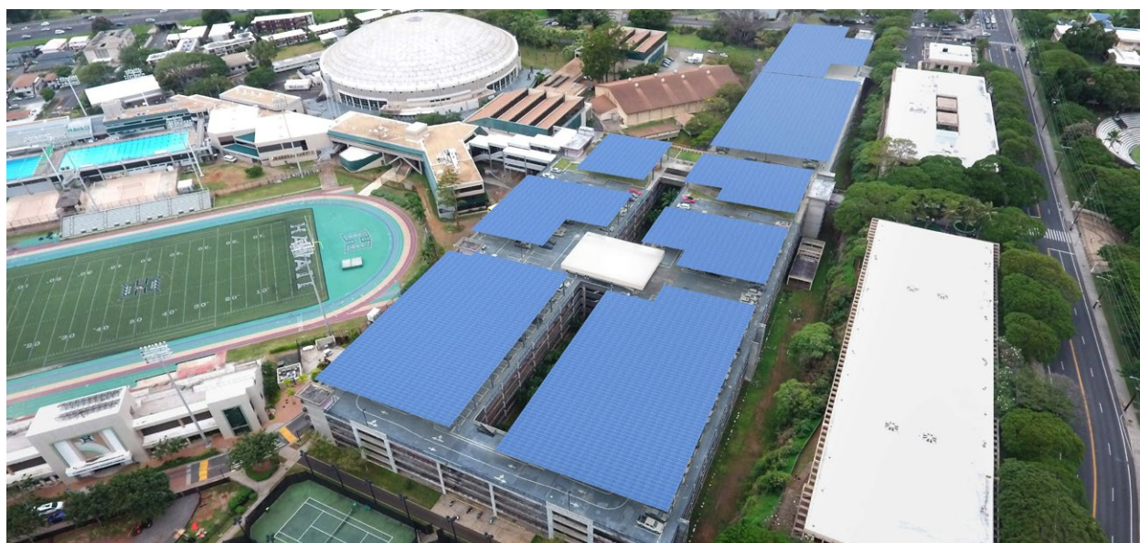
UHM parking structure PV installation
