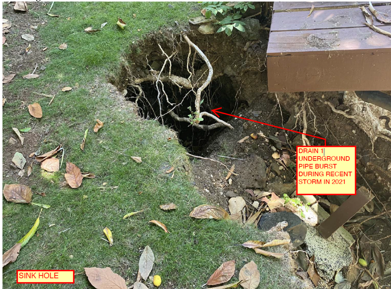
Figure 1: Photograph of Extensive Property Damage Resulting from City Roadway Discharge
