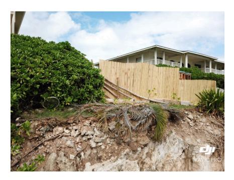
The hot tub below has been lifted up from its position onto the fire pit area, exposing grading on cliff surface inside the 40-feet shoreline setback. Other portions have further been terraced and leveled towards the ocean.
