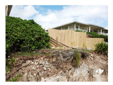
The hot tub below has been lifted up from its position onto the fire pit area, exposing grading on cliff surface inside the 40-feet shoreline setback. Other portions have further been terraced and leveled towards the ocean.
